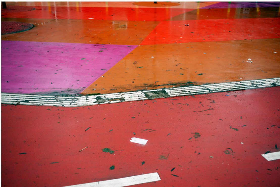
Indoor surface put outdoors, color fading, slippery when wet, frequently covered in grime
